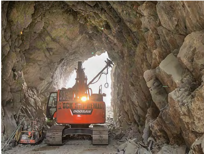
Daley-Rankin tunnel work.
